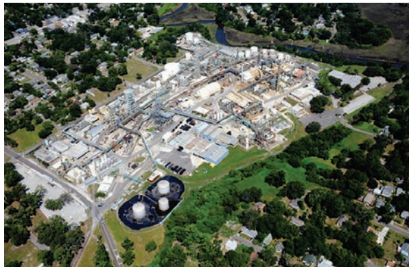
Two views of Renaissance's Jacksonville, Florida, facility
