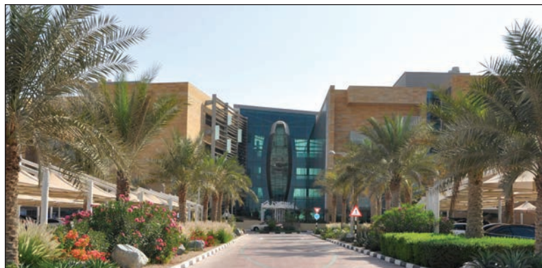
IFF's new flavor and fragrance facility in Dubai
