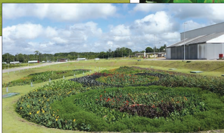
The Ecoparque, occupied by Symrise and Natura, employs “ecological industrialization” by using geothermal technology for air conditioning, while also using the site’s garden and lagoon system (pictured) to filter effluents.
